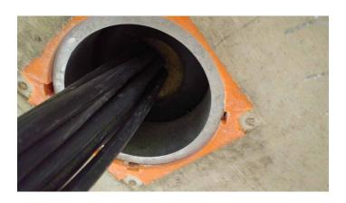
When the pipework is ready to be installed, remove the robust cap which is designed to provide a safe working surface until removed.
