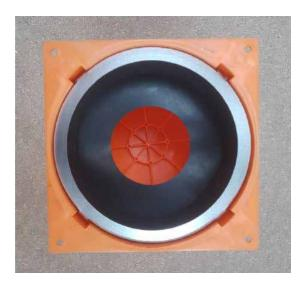
Job done! No extra work, backfill or sealant is required where the correct diameter pipe is used in the correct QuelCast. For QuelCast50 and where smaller diameter pipes are used inside larger collars then refer to the latter section of this
