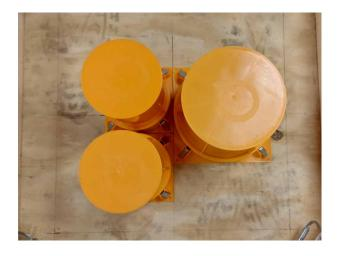
Fix the QuelCast to the formwork using suitable nails/screws through the preformed holes in the 4 corners.
